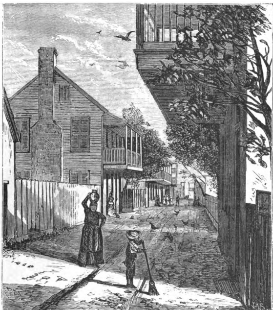
VIEW IN ST. GEORGE STREET.
